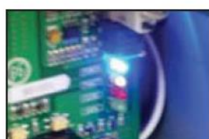
BOARD POWER ON LED SIGNAL CHECK
